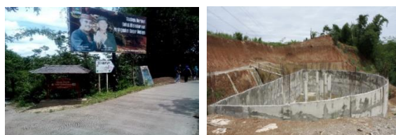
a. Concrete village road b. Construction of a stalled Museum
